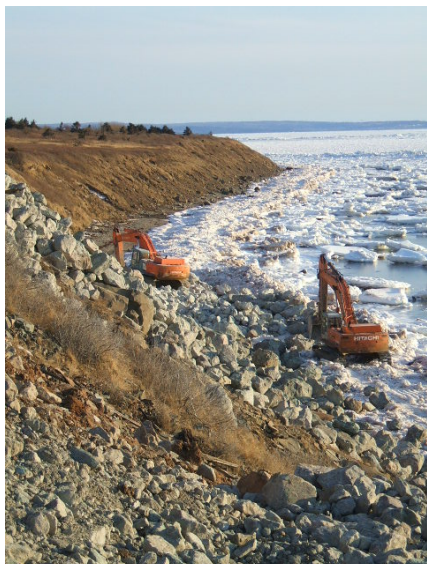
Coastal erosion prevention work.
