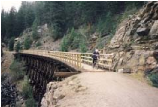
Myra Canyon Trestle in 2008 after rebuilding
