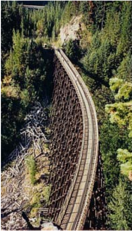
Myra Canyon Trestle 4 before 2003 fire
